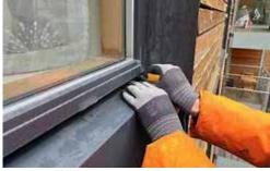
Water ingress above windows is often due to the fascia boards being incorrectly angled. They should be angled outward to direct rain water away from the unit.
